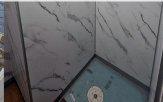
Bathroom: The wet room refurbishment was completed with new flooring, cladding, and enhanced lighting, creating a safer environment for the tenant.
